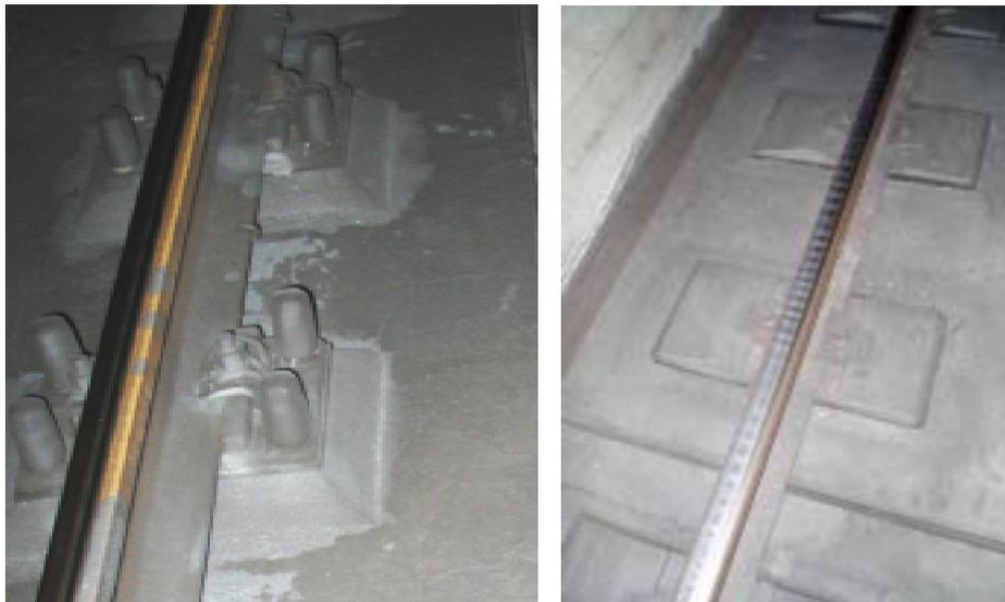
Figure 2. “Attacco tipo Milano” fastening system on “slab track” (left) and Nabla fastening system on booted sleepers on “floating slab track”.
