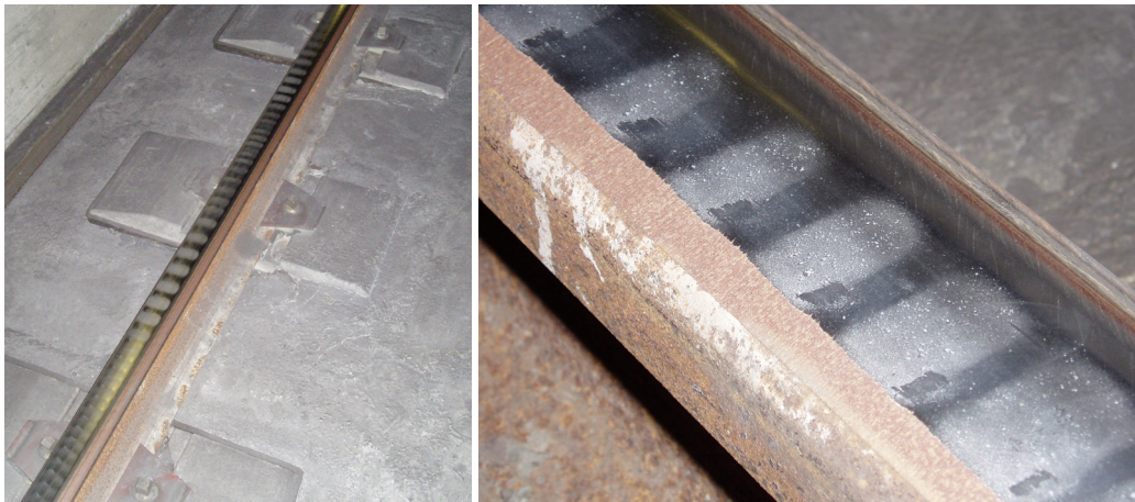
Figure 1: Rail corrugation appearance in a curve with floating slab track on Naples metro.
