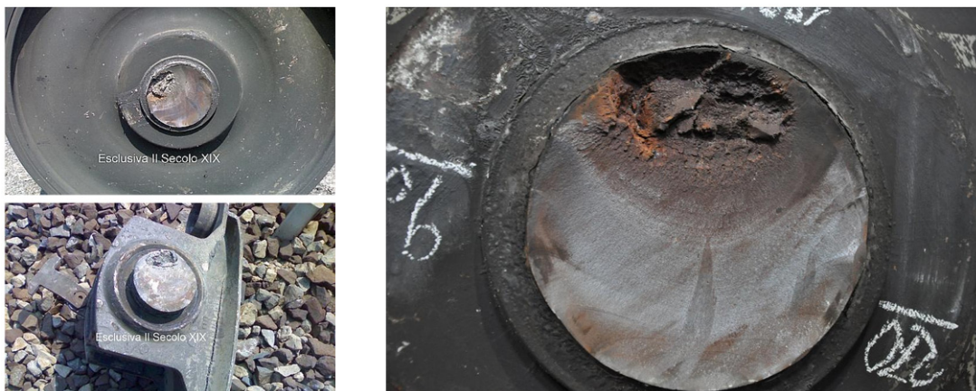
Figure 2: Axle broken in Viareggio as reported by the newspapers (left) and pictured during investigations after the accident (right).
