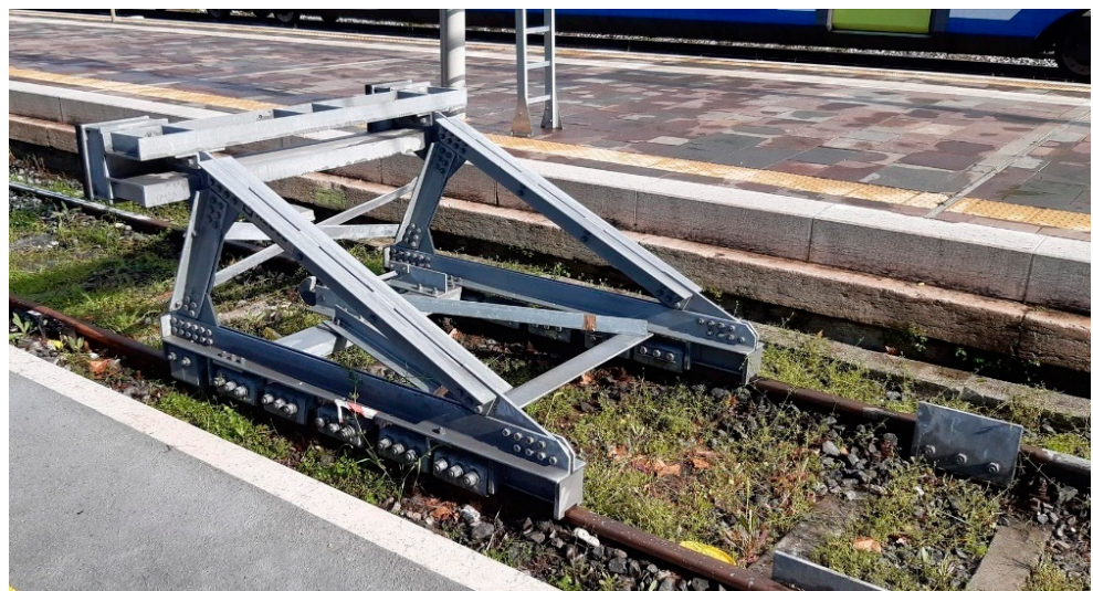
Figure 1. Example of a friction energy-absorbing buffer stop installed on a blind track in a station. (Photo by one of the authors).
